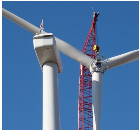
Construction of Pioneer Trail | White Construction
