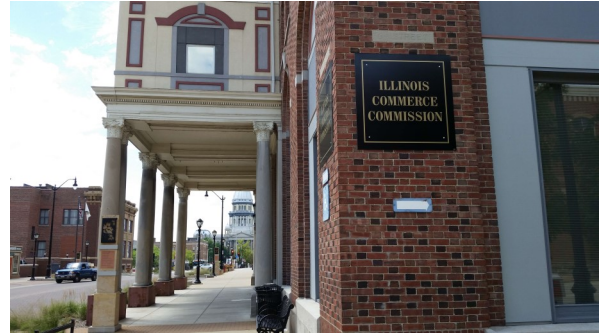
The Leland Building, headquarters of the Illinois Commerce Commission | ICC
