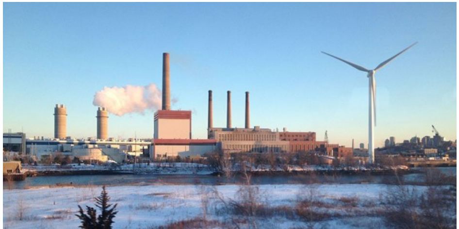
Mystic Generating Station
