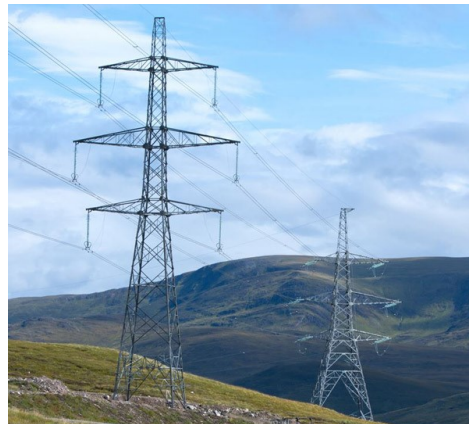
Transmission lines in Scotland | SSEN
